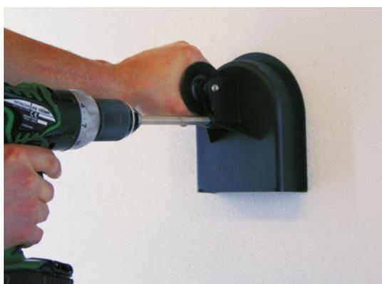
Press the bell-shaped firmly onto the insulating plate.
